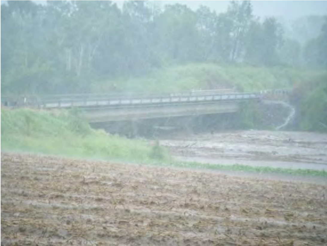
Figure 0.15. Zero minutes: Lockyer Creek at Kapernick's Bridge, 10 January 2011. (Source: Teresa Kluck).
