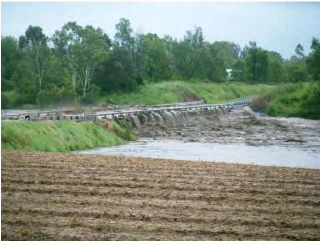
Figure 0.17. 20 Minutes later: Lockyer Creek at Kapernick's Bridge, 10 January 2011. (Source: Teresa Kluck).
