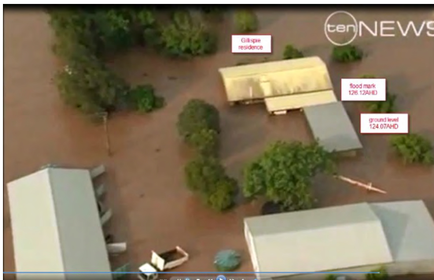
Figure 0.8. East of the quarry: note the depth of the flood as indicated by the muddy residue to the top of the house roof.
