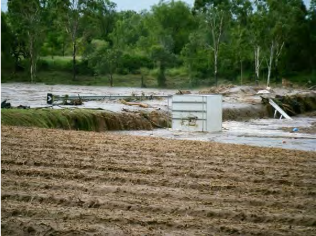
Figure 0.26. 100 minutes later: Lockyer Creek at Kapernick's Bridge, 10 January 2011. (Source: Teresa Kluck).
