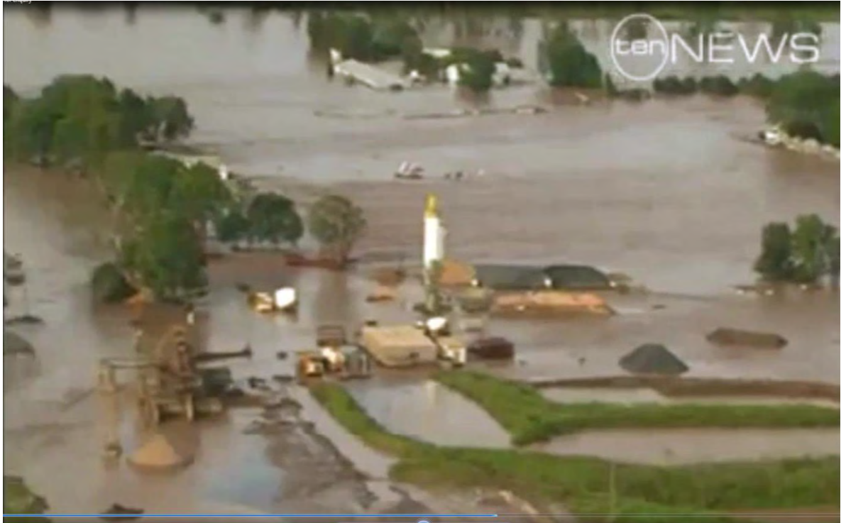
Figure 0.12. Video still: Sand batching plant at Grantham quarry. 10 January 2011. Note the piles of sand after the flood peak. (Source: Ten news aerial footage).
