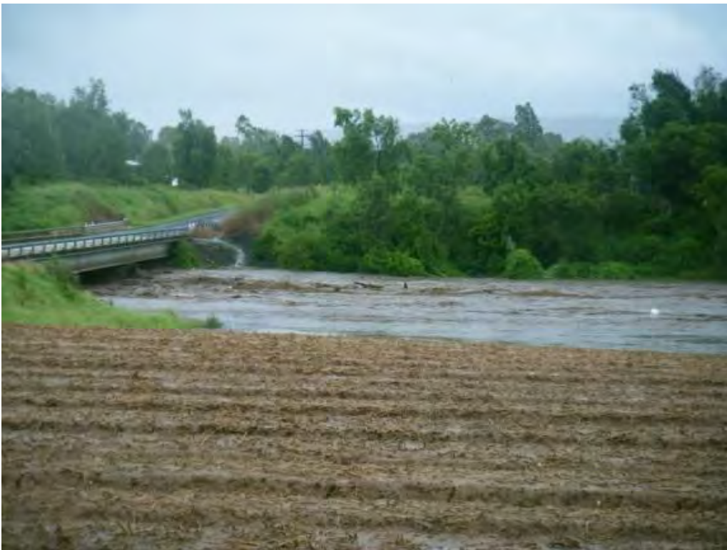
Figure 0.16. Eight minutes: Lockyer Creek at Kapernick's Bridge, 10 January 2011. (Source: Teresa Kluck).
