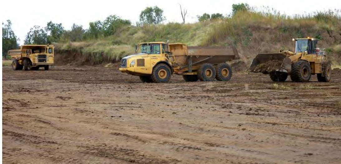
Figure 0.14. Grantham quarry. The same area as the aerial photo above. Note the height of the embankment compared with the dozer and trucks. (Source: The Courier-Mail)
