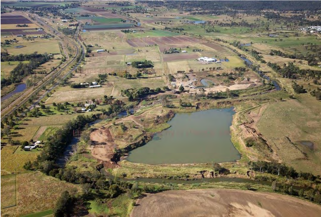
Figure 0.13. Grantham quarry: aerial May 2011. Note the area of earthworks on the northern side of the quarry where a section of remaining embankment is being taken away from what Denis Wagner claims publicly to be a ‘natural landscape’. (Source: The Courier-Mail)
