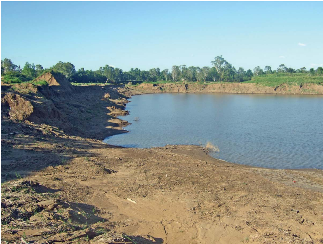
Figure 8.14 – Inside Western Levee Looking North as at 12 February 2011 (McIntosh 2015)
