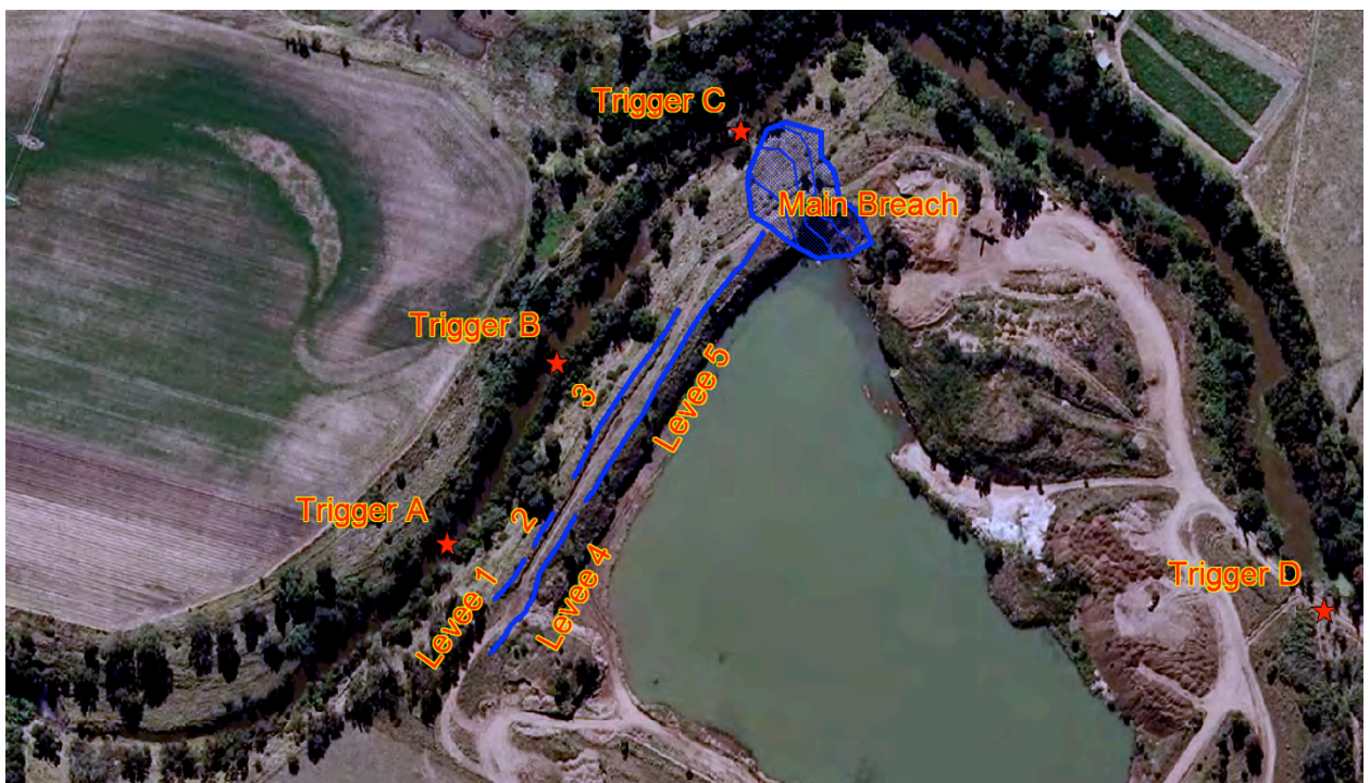
Figure 1.8 – Quarry Failure Trigger Level Locations
